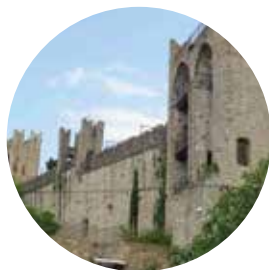
WALLS OF PIRAN
